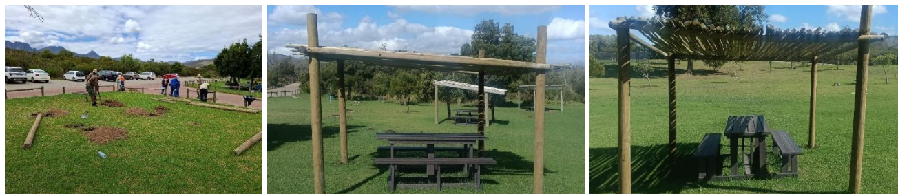
Figures 106 - 108: Shade structure construction and bench replacement at the HNR picnic area
