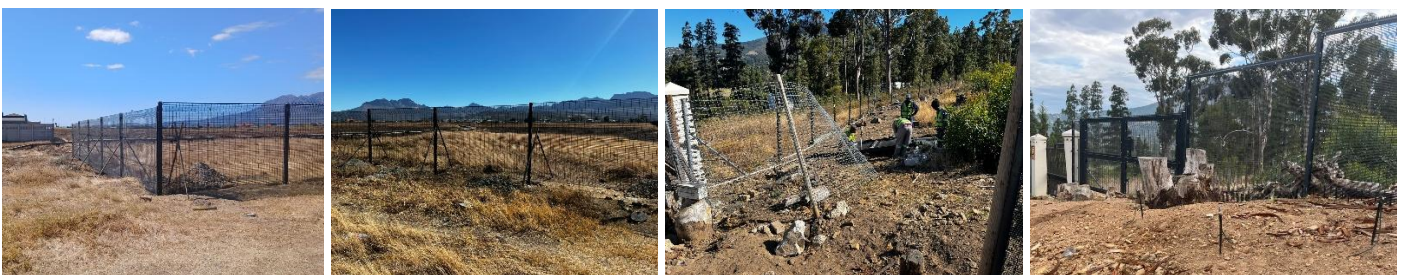
Figures 112 – 115: Installation of fencing at Harmony Flats & Schapenberg Nature Reserves
