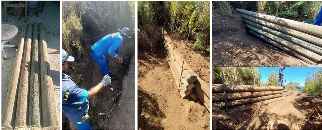
Figure 63 - 67: The construction of the water bar along White eye trail
