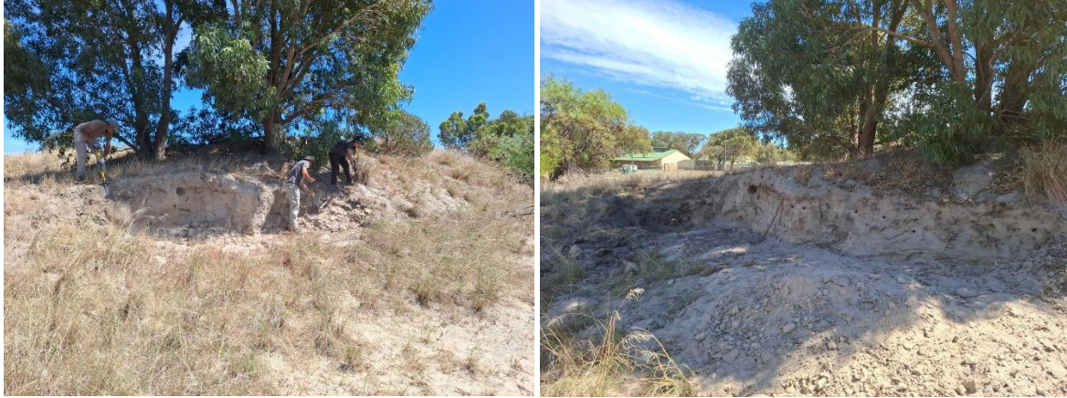
Figure 51: CSU staff cutting a dedicated nesting wall for European Bee-eaters. Figure 52: The finalized nesting bank at Paardevlei.
