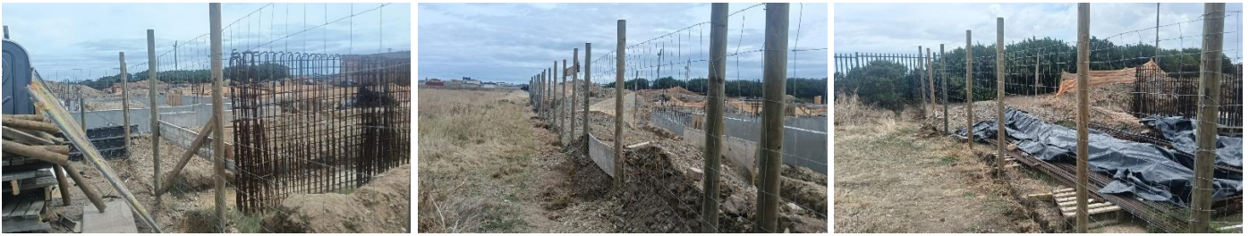
Figures 116 – 118: Temporary fence installation at Harmony Flats to secure the multi-purpose construction site following termination of the construction contract.
